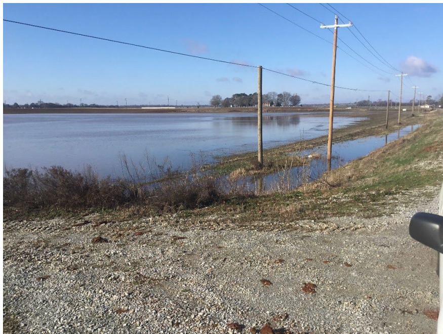
Image 5: Photo of the northern section of the Belle Mina Quarry site taken on February 12, 2024. After approximately 1.5 inches of rain on February 11, 2024, the property is completely covered with water and resembles a lake. This photo illustrates why this location is highly inappropriate for a limestone quarry or Sediment Basin 1. Photo by T.D. Murray facing southeast.
